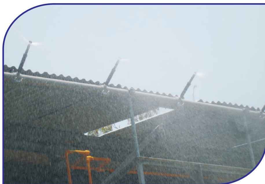
Fig.53 Automatic Fixed Water Sprinklers provided at CAL to absorb chlorine leaks
